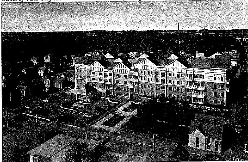
Oasis of Vine City under construction and part of the renewal and transformation of Vine City
