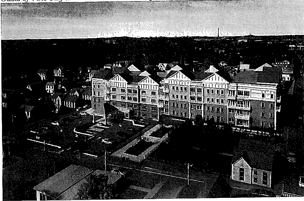
Oasis of Vine City under construction and part of the renewal and transformation of Vine City
