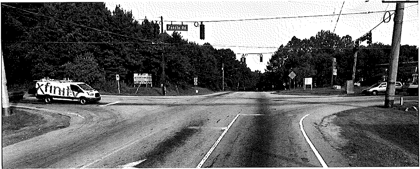
Photograph 1– Browns Mill Rd Facing West at Panola Rd
