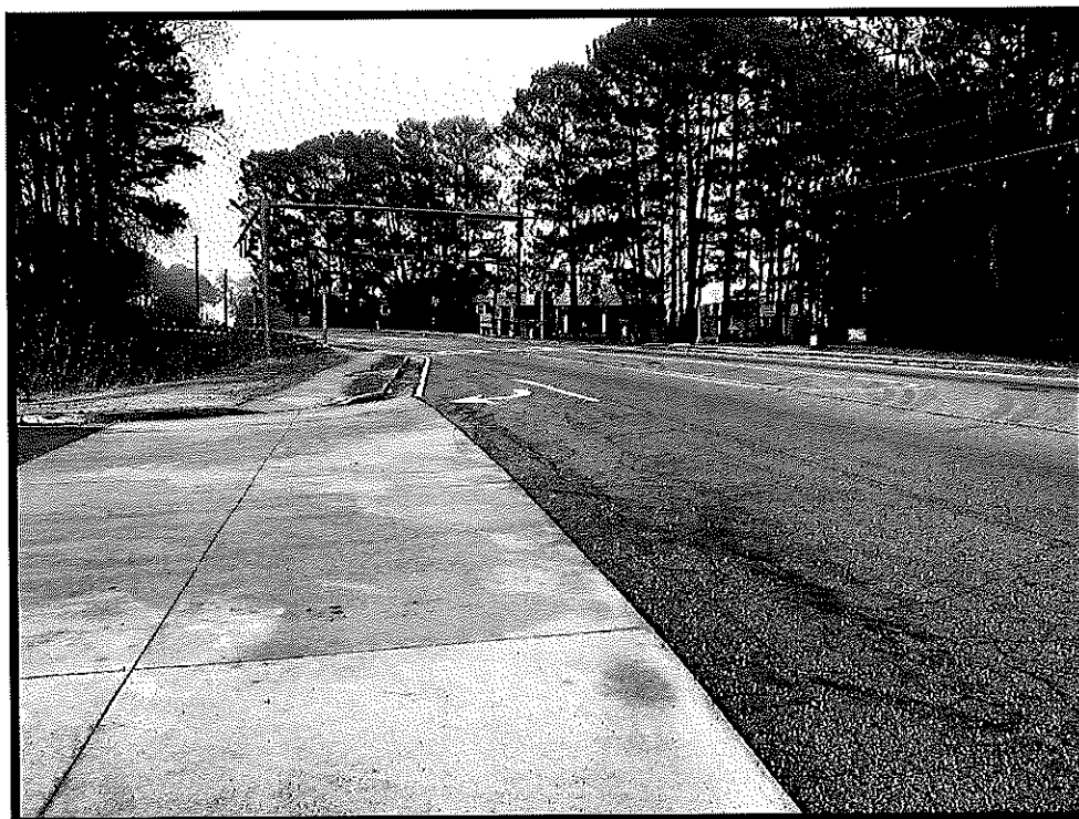
Photograph 6 – Fairington Road facing East at Chupp Way
